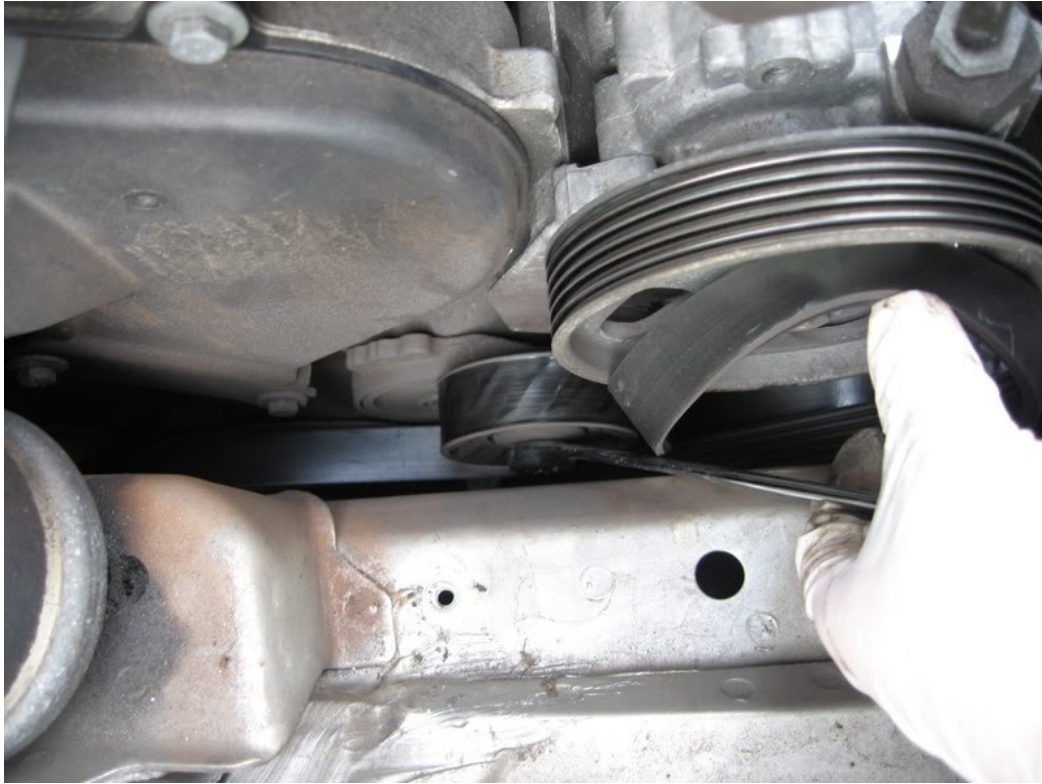
Belt being removed
